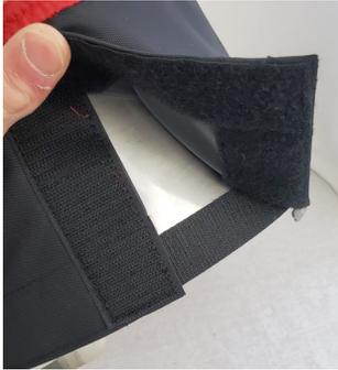
2. Unfold the fabric and open the velcro flap at the bottom. Fit the fabric around the duct, ensuring that the velcro strips on the bottom of the duct line up with the velcro strip on the bottom of the fabric. Finish installing the fabric by closing the fabric flap and lining up the velcro on either side of the flap.
